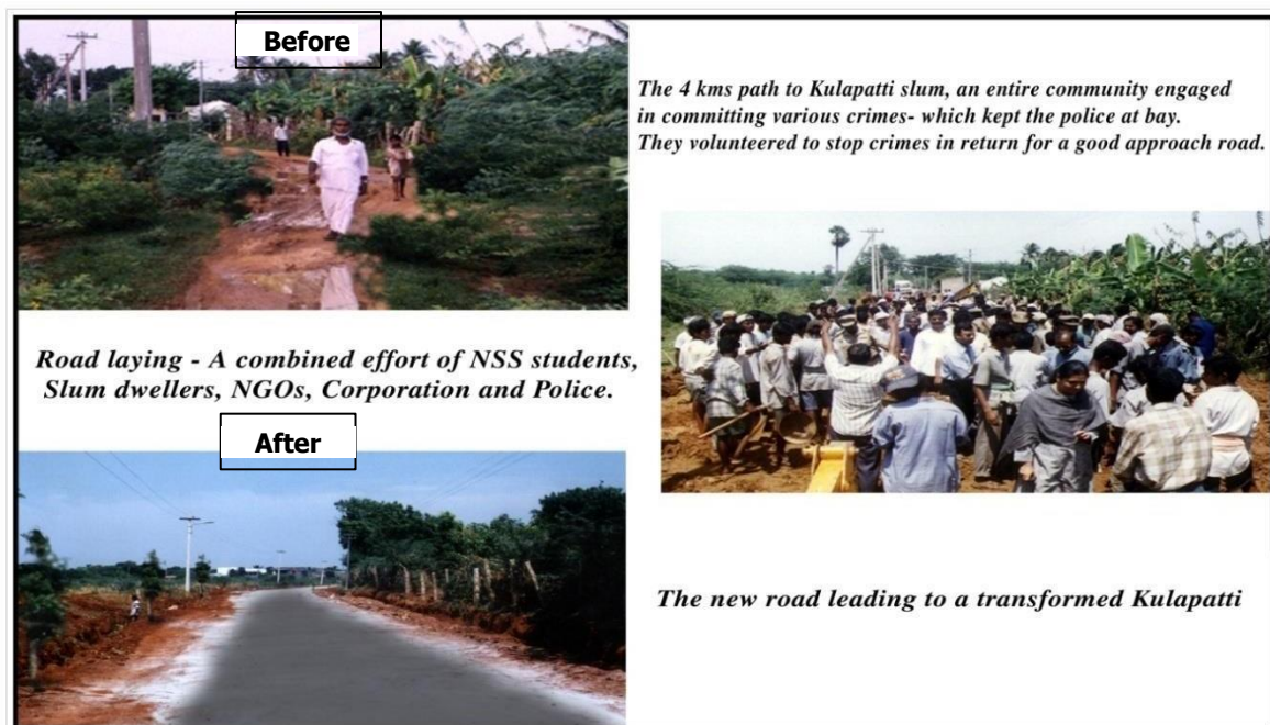
Image 8: Before and After Picture of Road Construction
